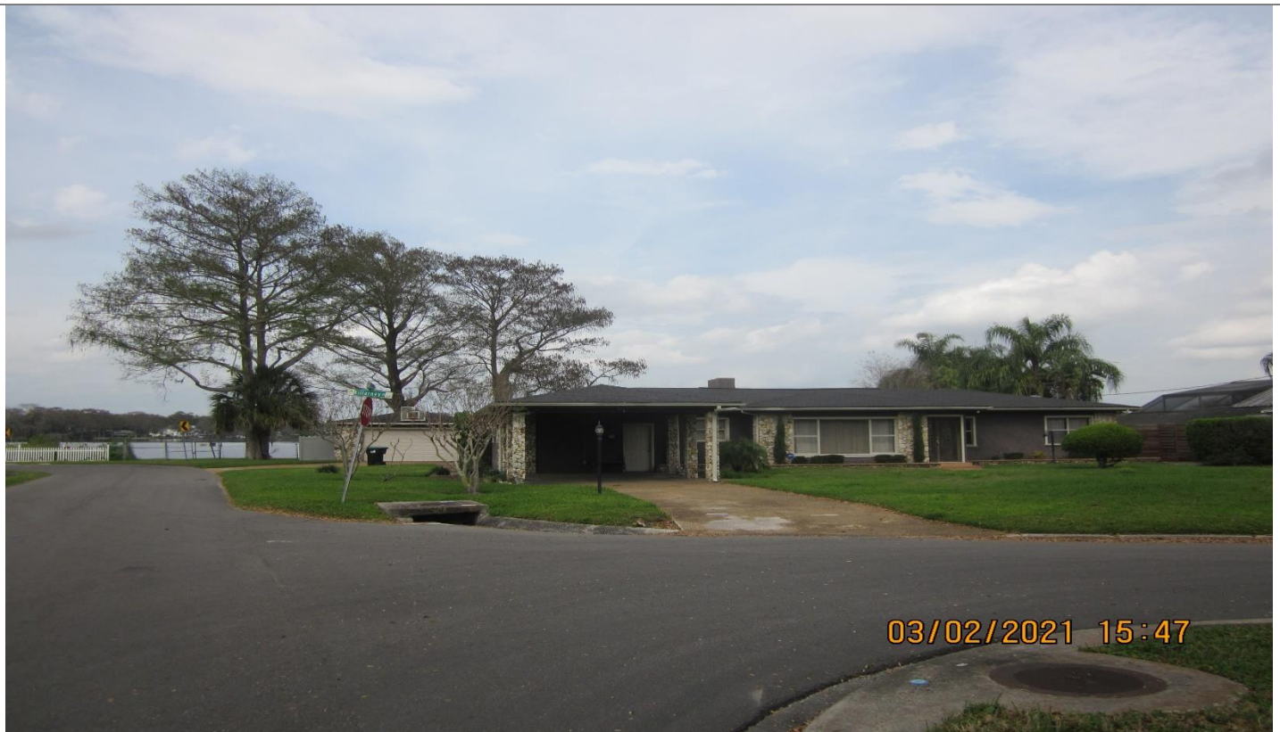
Subject property looking north to be demolished
