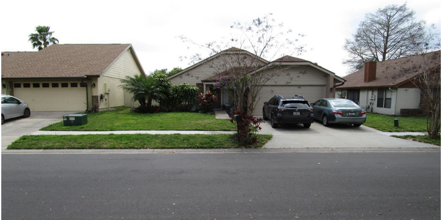
Front of property from Spring Valley Circle facing south
