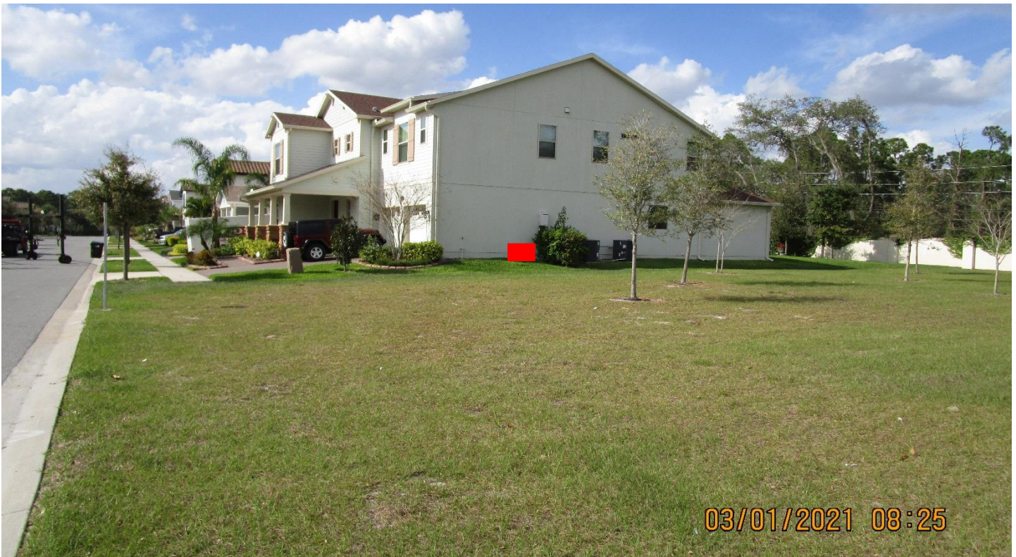
East side-proposed generator location facing west
