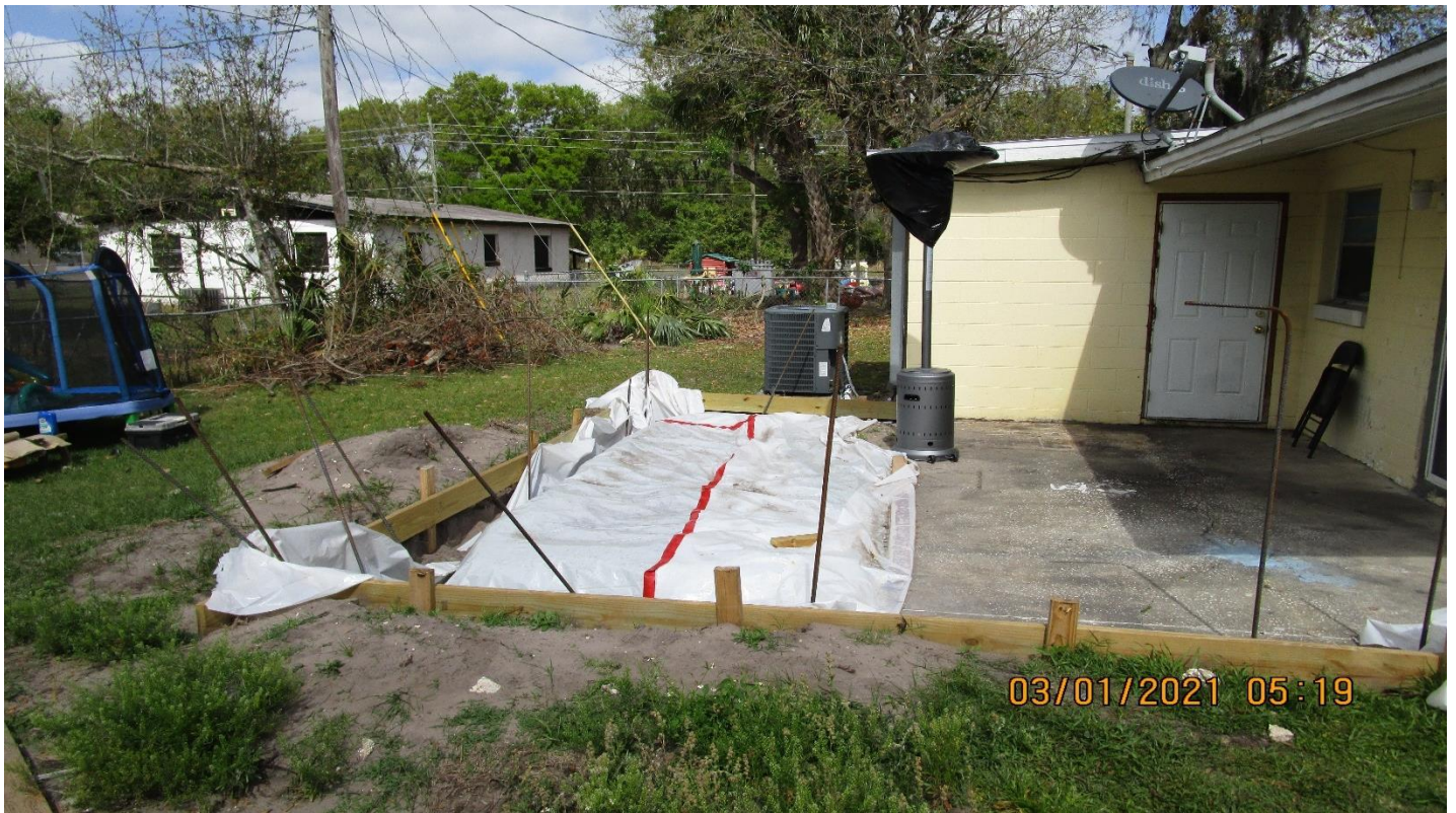
Location of addition facing north
