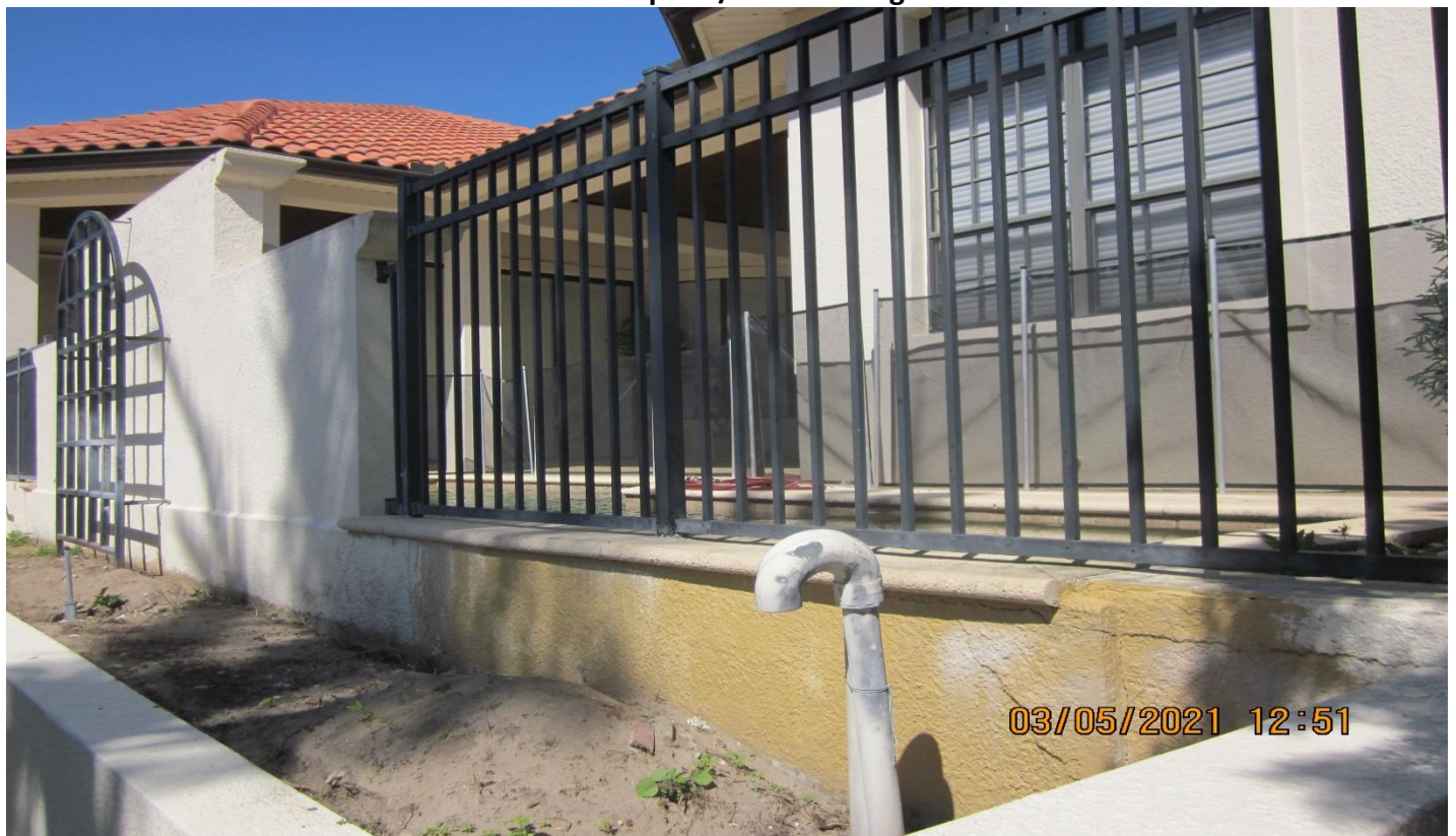
Planter and patio/lanai looking northwest
